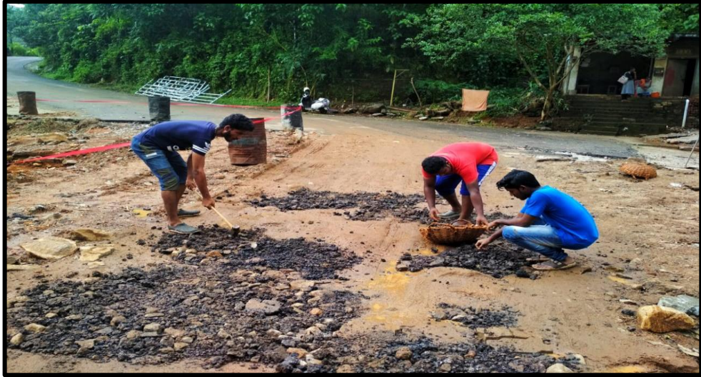
Road reconstruction after flood
