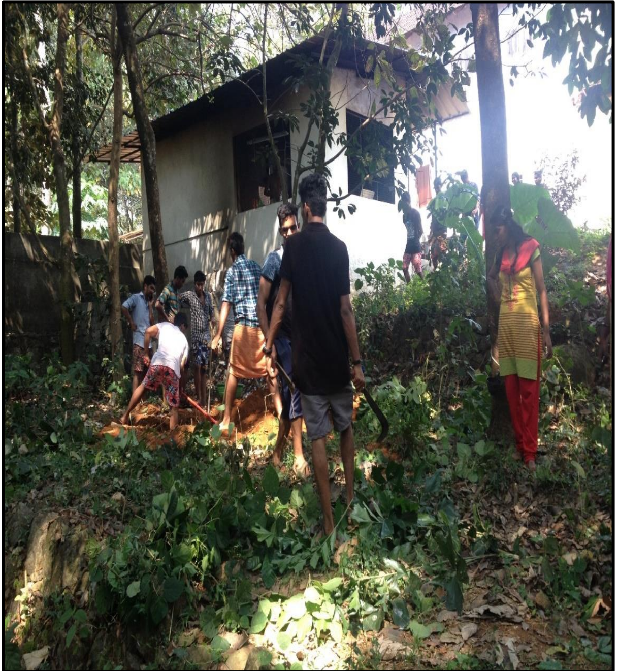
Constructing a rain water harvesting pit
